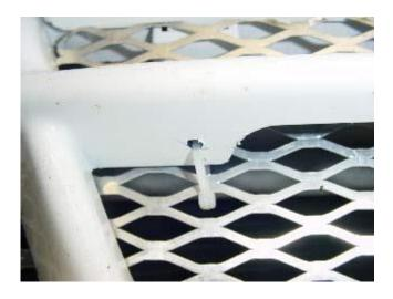
Just run the zip tie through the hole, around the mesh and tighten. Cut off the remaining length of zip tie. Do this for each hole that you drilled. If done correctly the zip ties are not visible from standing view.
